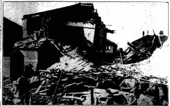
Wreckage at the rear of the house where casualties occurred.
