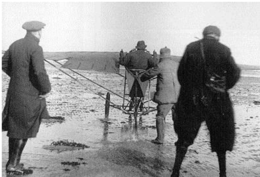
Above – Two pictures of ‘The Elsie’ at Littlehampton after it had been altered to have a wider undercarriage. xxxiii
